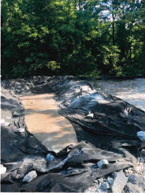
5/20/2024 Inside berm after cleanup with new fabric
