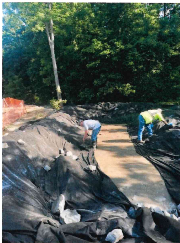
5/20/2024 Replacing filter fabric
