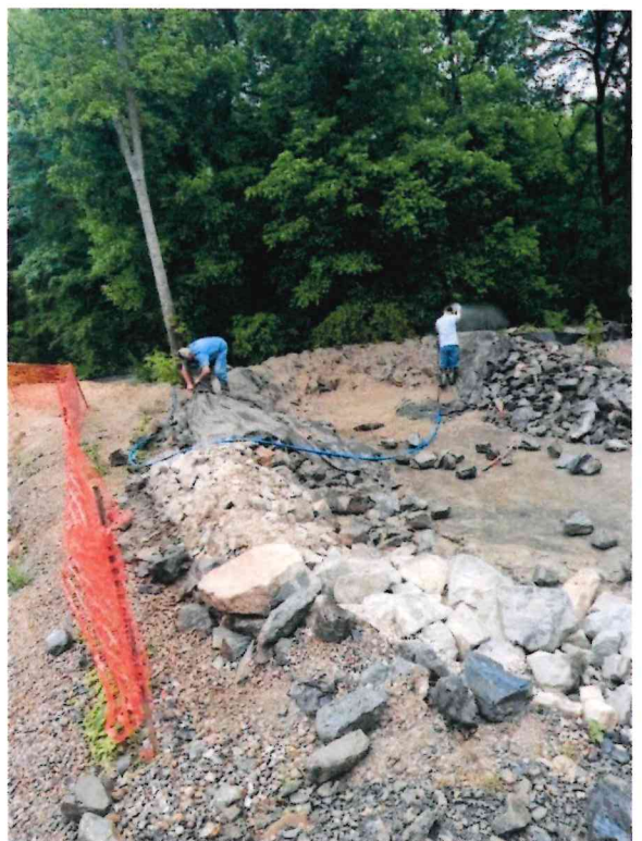
5/13/2024 - Inside berm during cleanup and replacement of filter fabric
