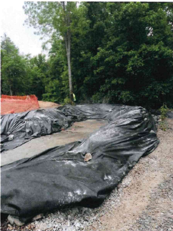
5/13/2024 - Inside berm after cleanup with new fabric
