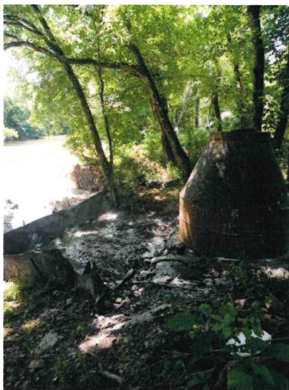
May 28, 2024 - MH 1748 after cleanup with new silt fencing
