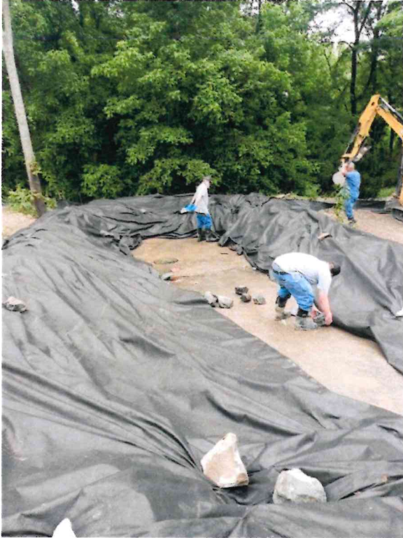
5/13/2024 - Replacing filter fabric
