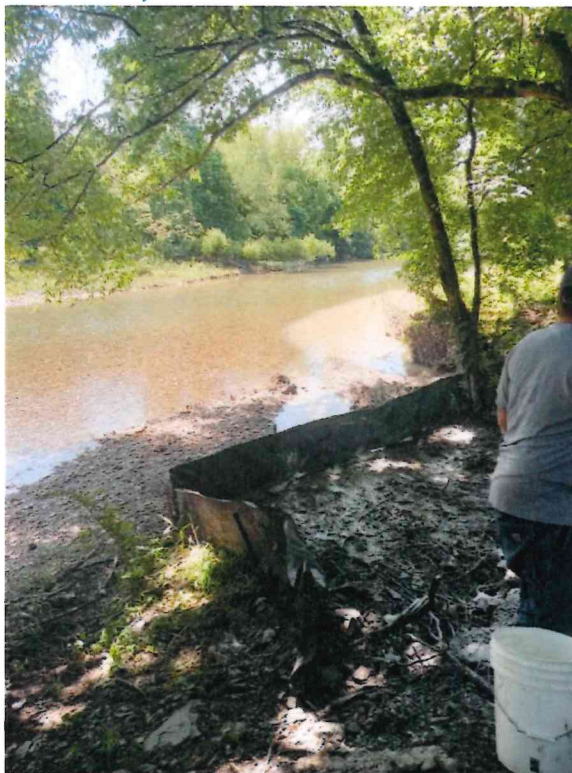
May 28, 2024 - MH 1748 after cleanup with new silt fence
