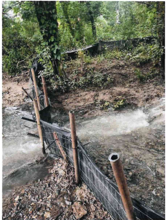
May 5, 2024 - Stabilizing silt fencing
