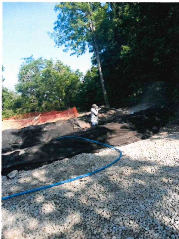
5/20/2024 Inside berm during cleanup and replacement of filter fabric
