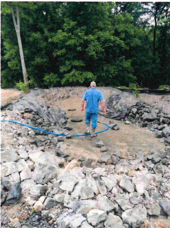
5/13/2024 - Inside berm during cleanup and replacement of filter fabric
